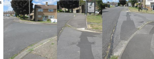
Drop-kerbs. First image is Bingham Road and Bishopdown Road by Catholic Church, very poorly done. Second & Third are upper entry of Hoadley Green, the drop-kerb is only applied to one-third width of the pavement, it stands proud of the road, the surface of which is poor.
