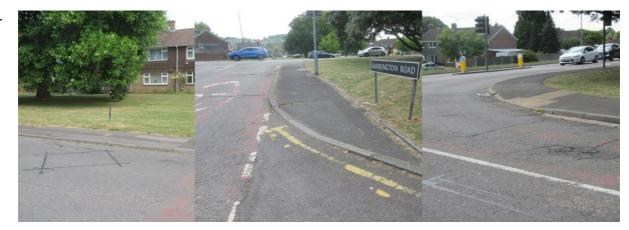
Barrington Road road-sign completely missing, apart from one post. Drop-kerb to access London Road pavement is very poor. Drop kerb from London Road crossing the entrance of Barrington Road is also very poor for wheelchair users.
