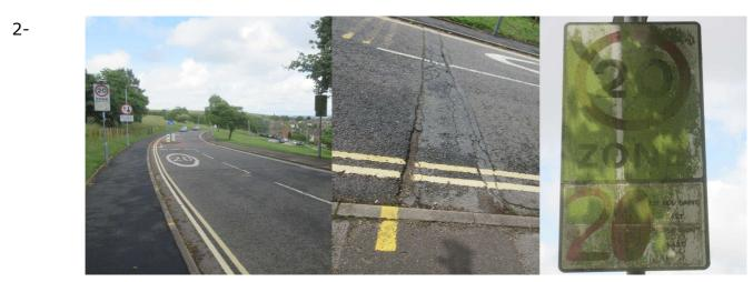
Entry of 20mph zone, top of Bishopdown Hill. The 20mph sign is filthy, mostly due to being close to tree overhang. Adjacent to it a trench in the road needs filling again.
